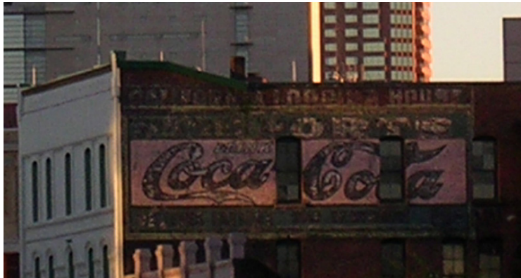
End of an era: The faded green and white Coca-Cola sign on the former California Lodging House disappeared under black paint on the afternoon of August 14, 2006. Now a plastic billboard promoting the Make a Wish Foundation has taken its place on the north wall of the building at 207 NW Third Avenue.
