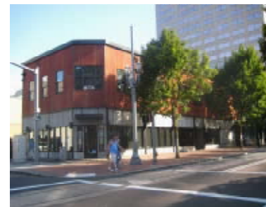
Roseland Theater renovations
