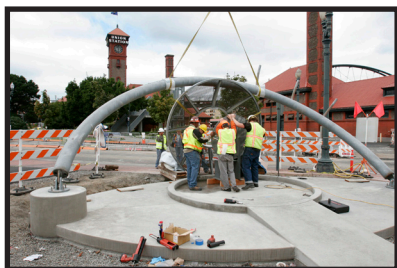
Construction continues near Union Station
