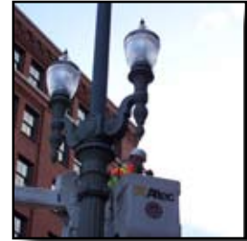
Ornamental street lights are being installed in the North Mall
