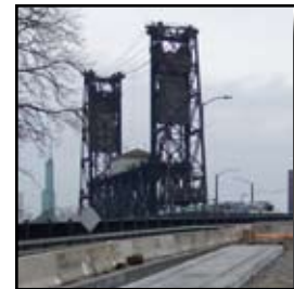
New light rail tracks approach the Steel Bridge
